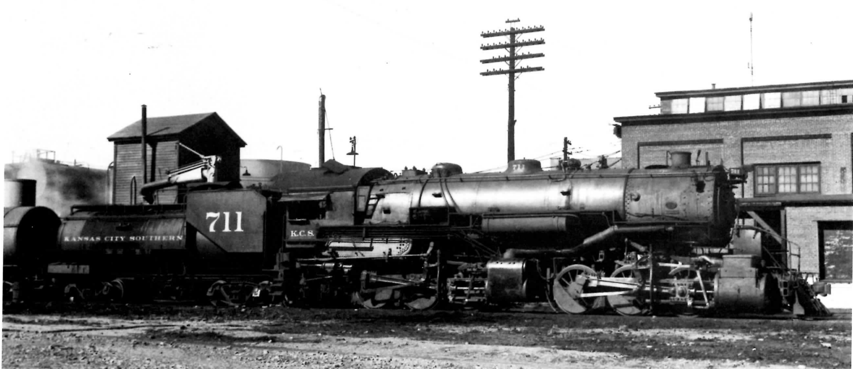
The 700 series 0-6-6-0 Mallets were unusual road power. 700 (above), on the Watts, Okla. turntable circa July, 1924, was in helper service north from there. 711 (below), at Shops, La., February 11, 1940, takes on oil before leaving with the Leesville local freight.
