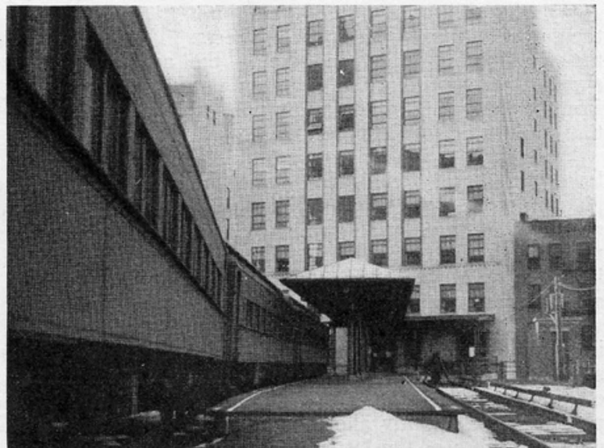
Here Is a Strange Station Combination. The Yonkers (N. Y.) Terminal of the New York Central's Putnam Division Is Located at the Third Story of the City's Leading Bank
