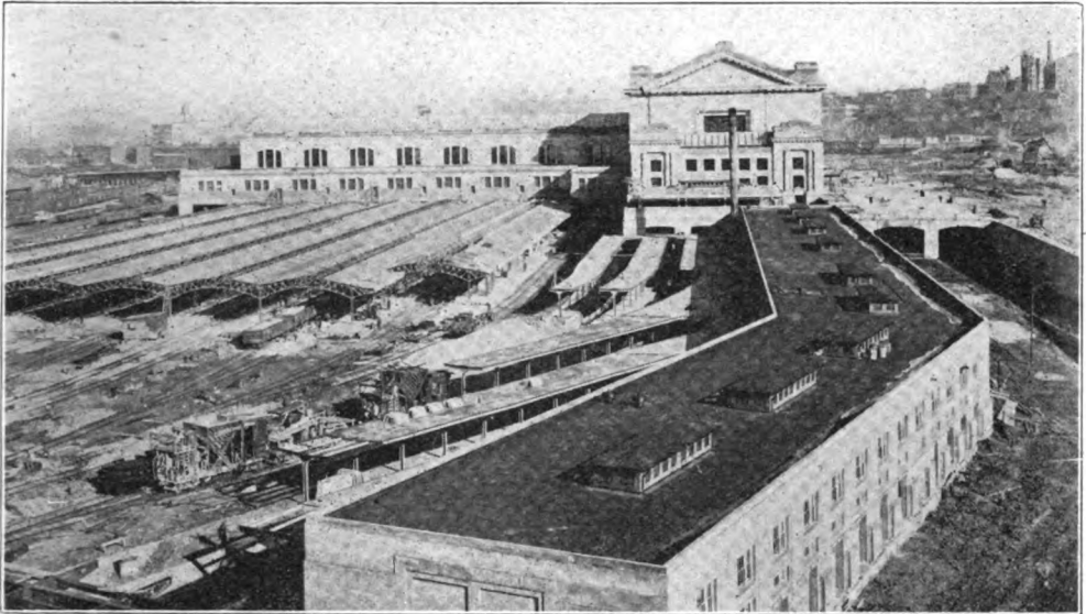
FIG. 4.—WEST VIEW OF STATION, SHOWING EXPRESS BUILDINGS, TRAIN SHEDS AND WEST EXPOSURE OF MAIN BUILDING AND WAITING ROOM.
