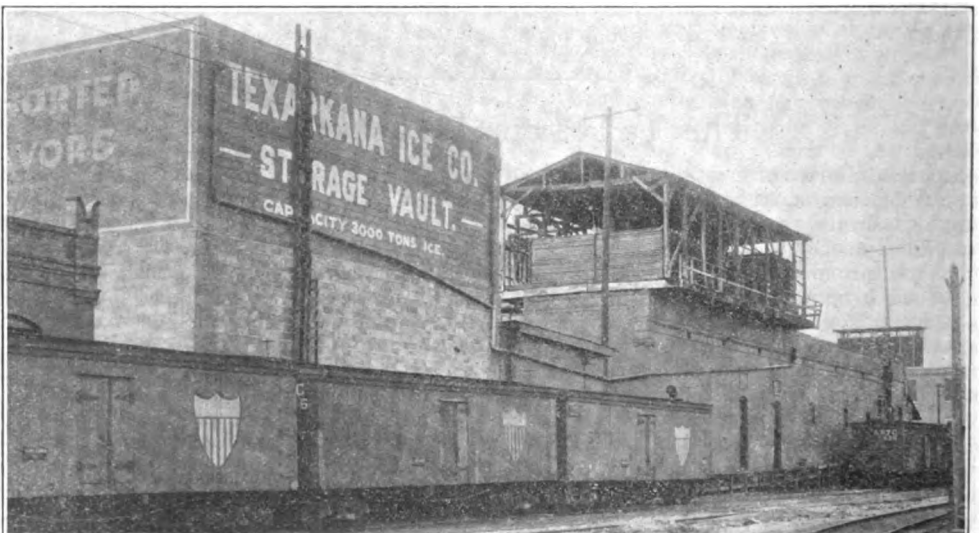
TEXARKANA ICE COMPANY'S COLD STORAGE PLANT.
