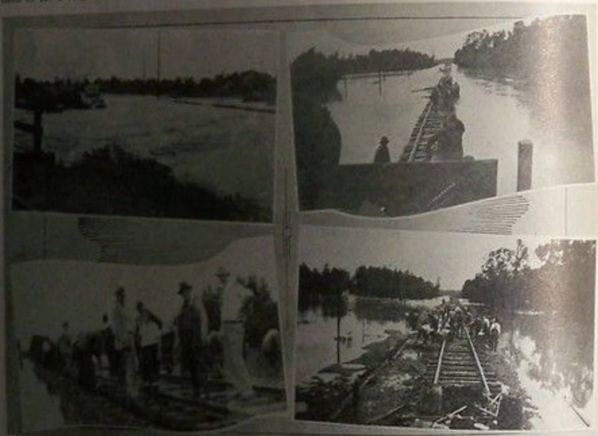
Scenes during the high water south of Texarkana on Sunday, May 18. The view at the upper left was taken late that afternoon from the end of bridge B-296. At the upper right is a view on Mile 489, and below it, another view in the same vicinity. At the lower left is a group of Texarkana employees at the washout.
