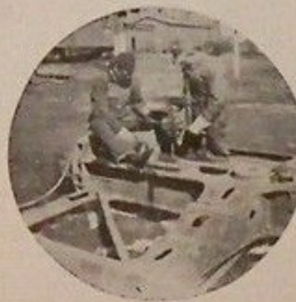
Drilling Steel Underframes, Pittsburg Shops
